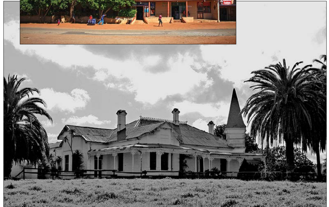
One of the finest examples of grand Victorian/Edwardian architecture in the region, Schoonspruit is situated just south of Malmesbury facing the old road north
