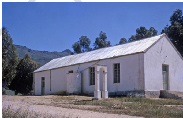
The Sendingkerk in Riebeek Kasteel before demolition.
